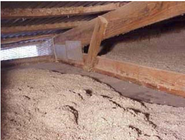
Growers should inspect the attics of their houses at least once a year. While in the attic they may notice that insulation has been blown around by the wind. Moved insulation can cause sweating and therefore deterioration of the house.
