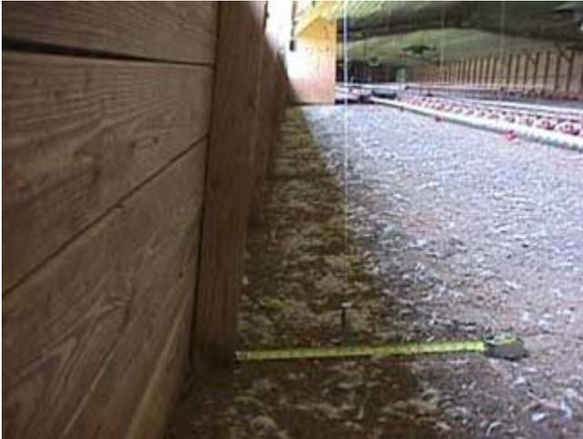
The posts in this poultry house were not set deeply enough in the ground. Because of the shallow embedment depth, this wall is leaning almost a foot. This type of structural problem is difficult to fix. It will definitely shorten the life of the poultry house.
