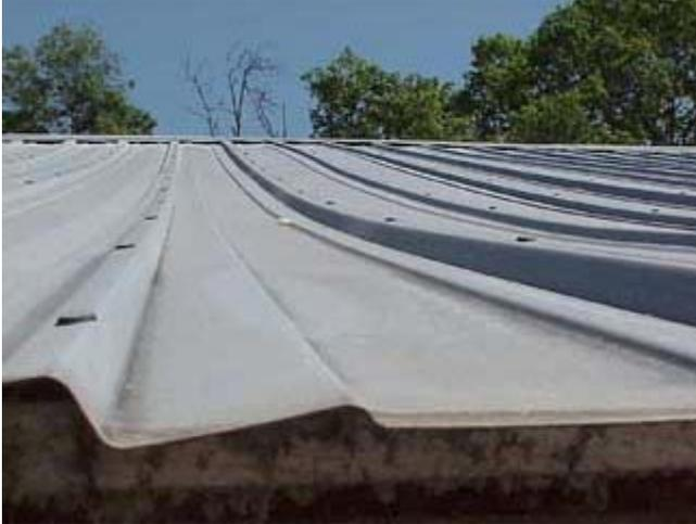
From a distance the ridge line of this house looks straight and the house appears to be in good shape. Looking closer, however, you can see serious sagging in the roof framing of this house. This house has center rows of posts. Removal of the posts and replacement with a modern truss will not correct this sagging. It is questionable whether houses with sagging roofs should have extensive upgrades made to them.
