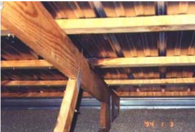
This shot in the attic of a relatively new house shows that there is a roof leak near the second purlin. A nail or screw probably was misdriven. If this leak is not repaired the truss will be rotted and the purlin will break, causing a serious structural problem. An attic inspection during a light rain is an excellent way to find these deficiencies.
